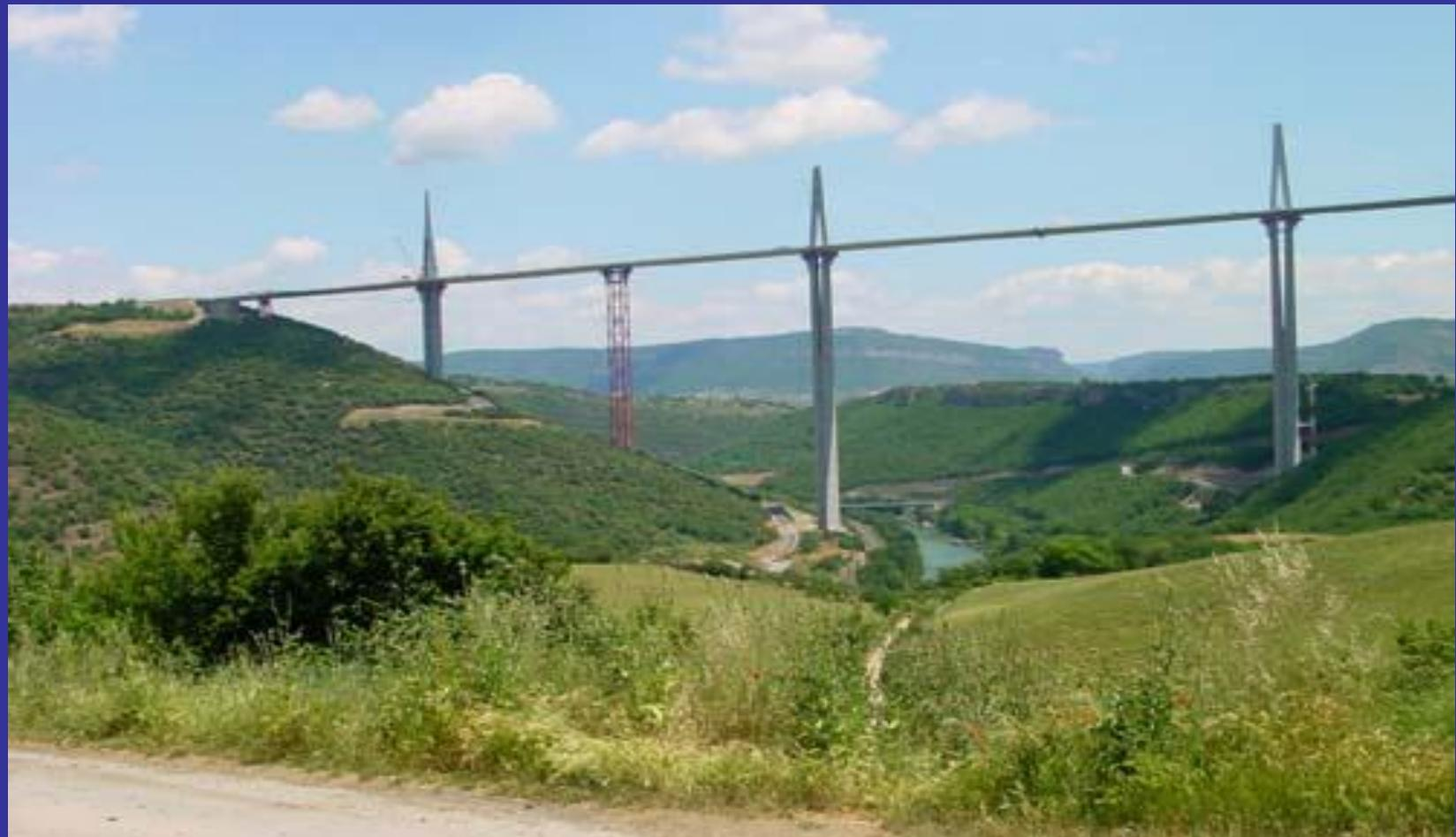
This suspension bridge has a total length of 2.5 km and crosses the Tarn River. It is 343 meters high, a world record. The road, with two lanes on each side, will cross the river at 270 meters above ground. At its highest point, the viaduct is even higher than the Eiffel Tower. Conceived by Norman Foster, this suspension bridge is supported by seven pylons, instead of the two that are common for this kind of construction.
